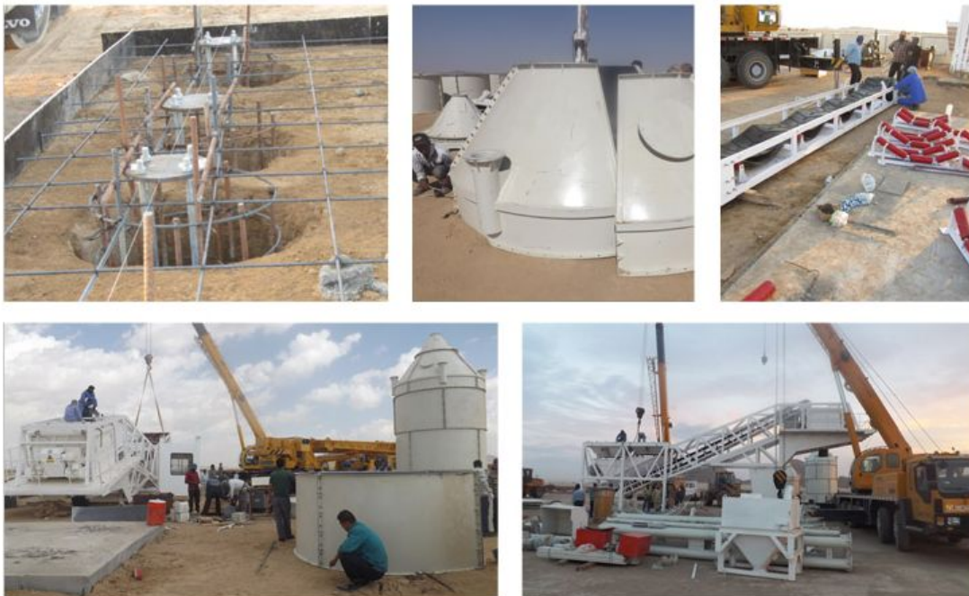
Installation of YHZS60 mobile concrete mixing plant
